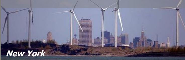
Wind turbines installed during remediation at abandoned steel mill
