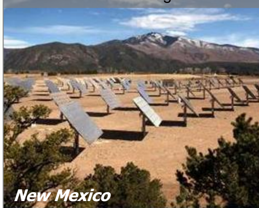
Concentrators installed on remediated mine tailings
