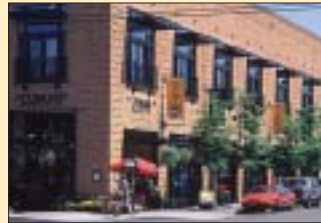
1 Portland, OR: By recycling the long-vacant “Old Carnation Dairy” into a high-density, mixed-use, energy-efficient housing and retail development, Portland and its private partners have helped revitalize the City’s Sunnyside neighborhood and Belmont Business District.
