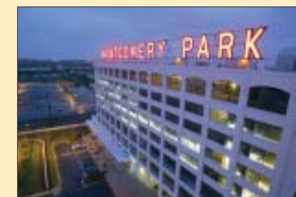
6 Baltimore, MD: The former east coast distribution center for Montgomery Ward is now a 26-acre “green” redevelopment that has leveraged over $60 million in private investment, will generate over 3,000 jobs, and is the new home to the Maryland Department of the Environment.
